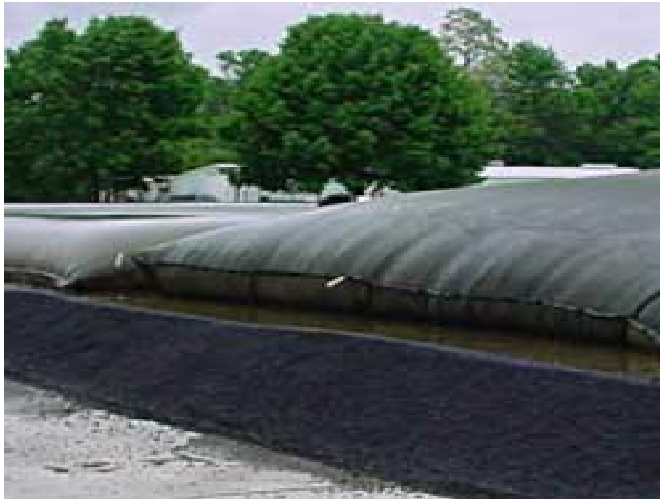
Geo-tubes used for dewatering sediments from the Upper Sheboygan River, 2007
