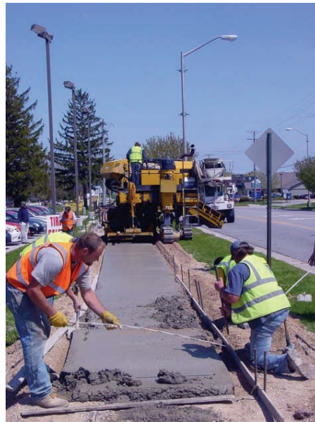
Eastern Avenue Sidewalks, Plymouth Looking East (During Construction)
