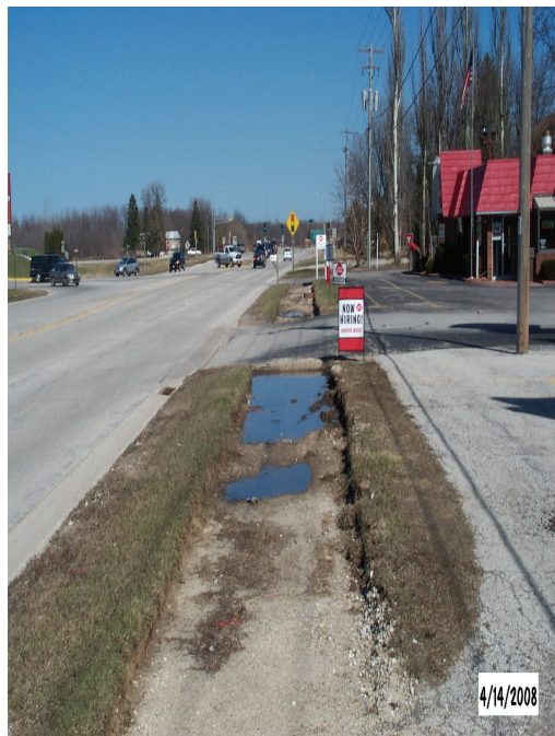
Eastern Avenue Sidewalks, Plymouth Looking East (Before)
