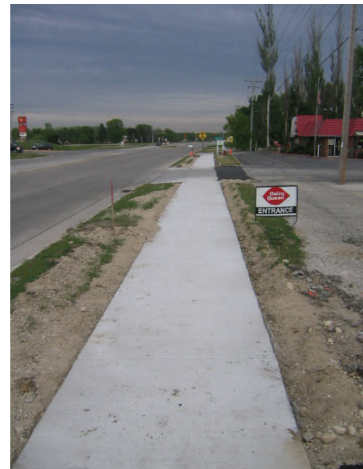
Eastern Avenue Sidewalks, Plymouth Looking East (After)
