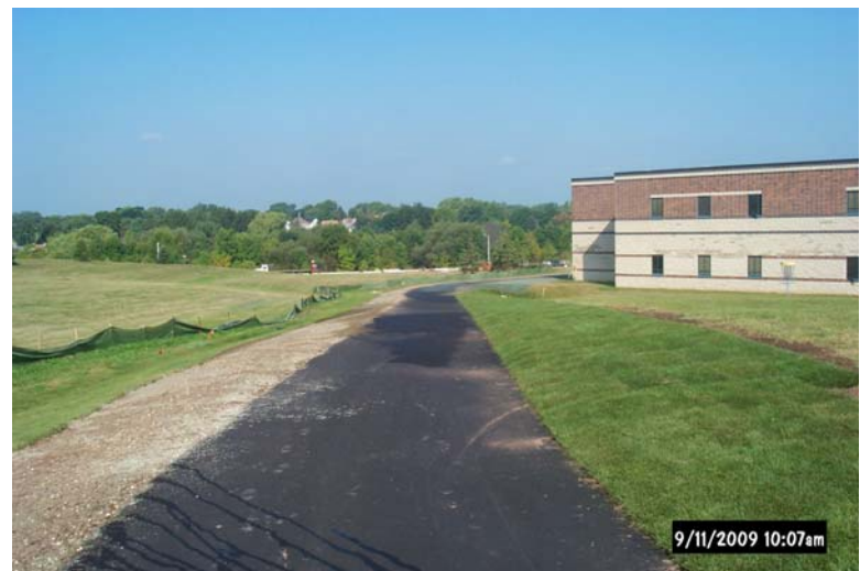
High School Playfield Entrance (After)
