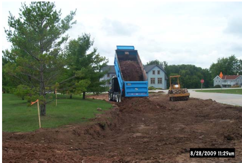
High School Entrance Looking West (During Construction)
