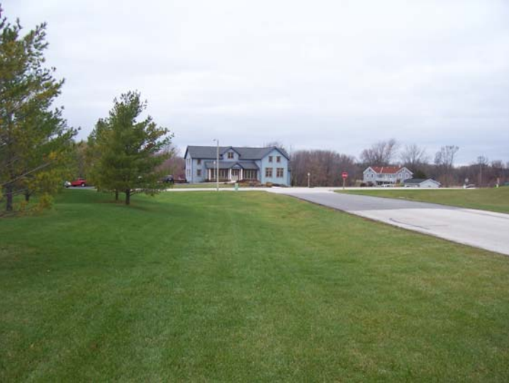
High School Entrance Looking West (Before)
