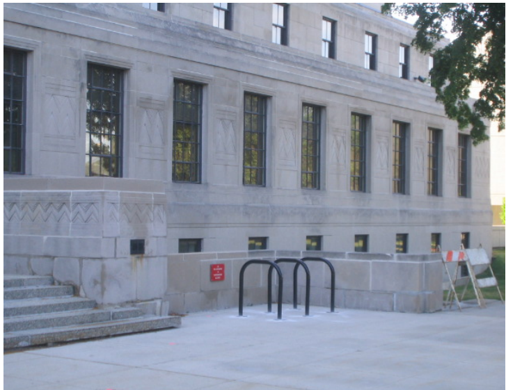
After a long wait, the racks are finally installed at the County Courthouse.
