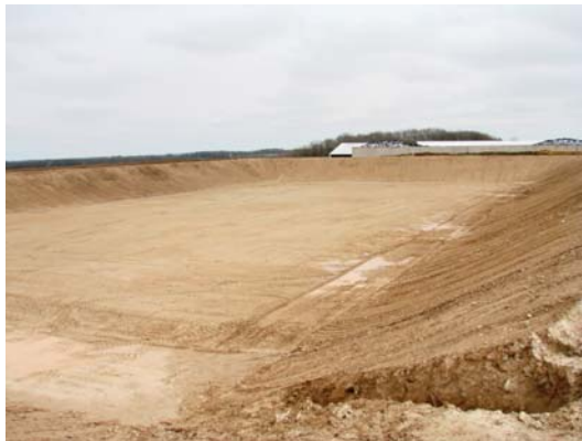
Excavated Liquid Storage at Drake Dairy, Inc. Ready for Concrete Liner 2008
