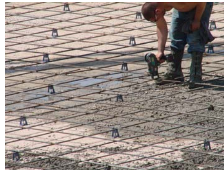
Steel Placement/Tying Prior to Pouring Concrete Liner at Drake Dairy, Inc. 2008
