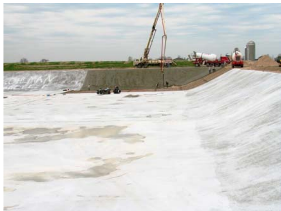
Last Concrete Pour of Liquid Storage Facility at Drake Dairy, Inc. 2008
